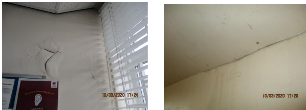
Figure 7 – Water and damp in the consulting rooms
