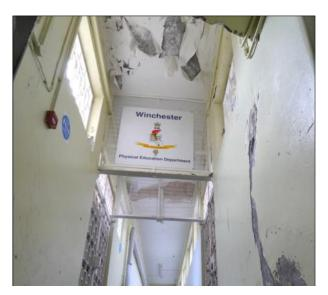
The ceiling in the staff toilet in reception leaks and the staff have rigged up a framework of broom handles and plastic to remove water (right).
