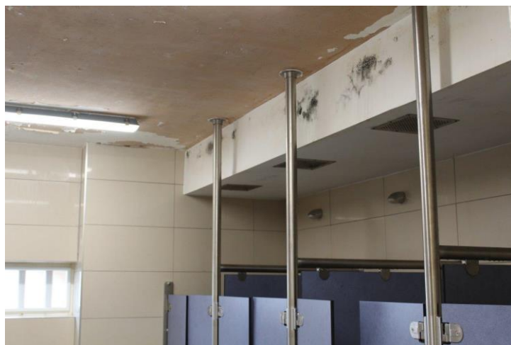
Mould and peeling paint in a refurbished shower room
