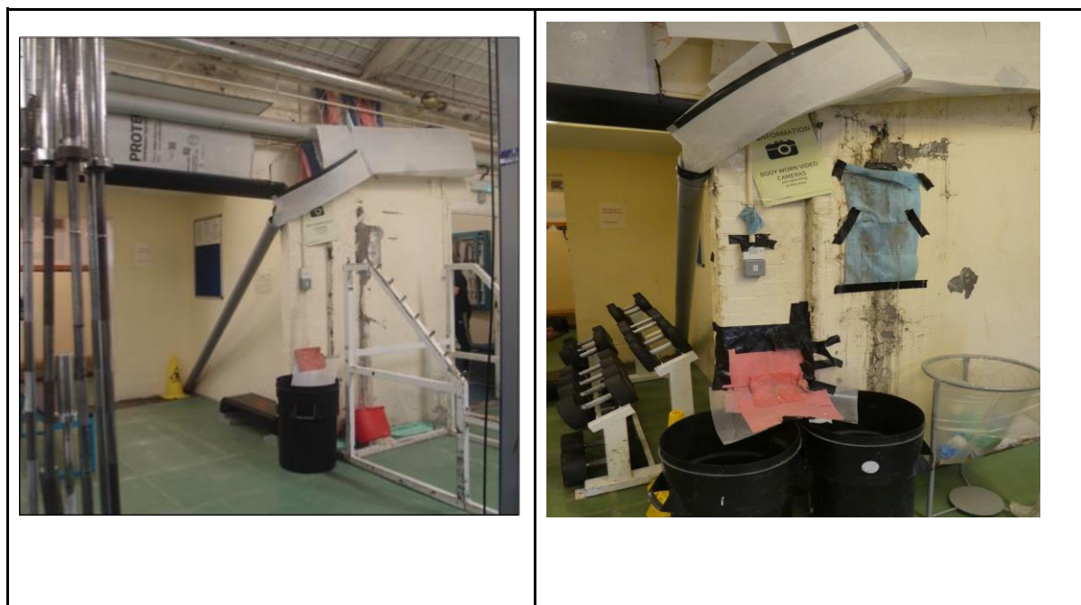
Photo 3: water ingress damage in the gym in May 2023 and continuing in May 2024.
