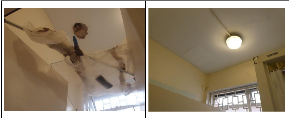
Photo 2: the ceiling in the reception staff toilet has been repaired (before and after photos)
