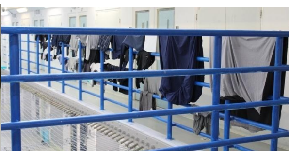
Fig 6. Clothes drying due to broken dryers
