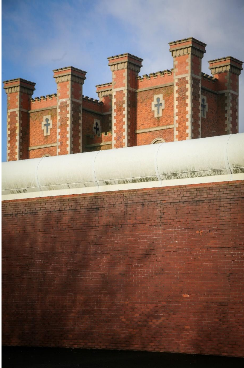
Original prison façade, seen behind the modern outer wall (Image: © Andy Aitchison)
