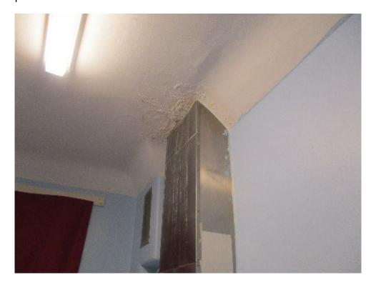
Induction cell with damp on the ceiling
