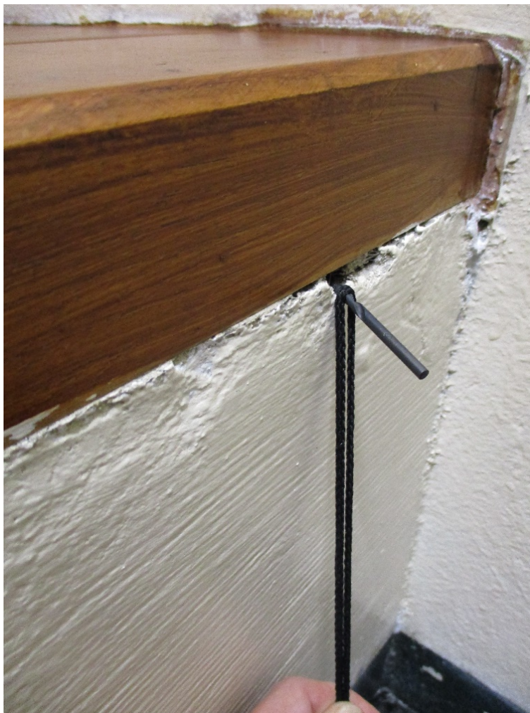
Potential ligature point under a bench at Croydon Magistrates' Court
