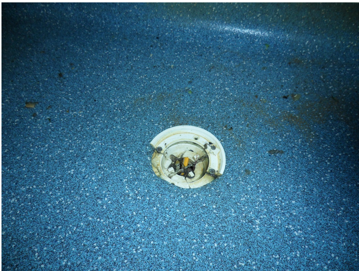
Damaged and dirty drainage sink in shower area
