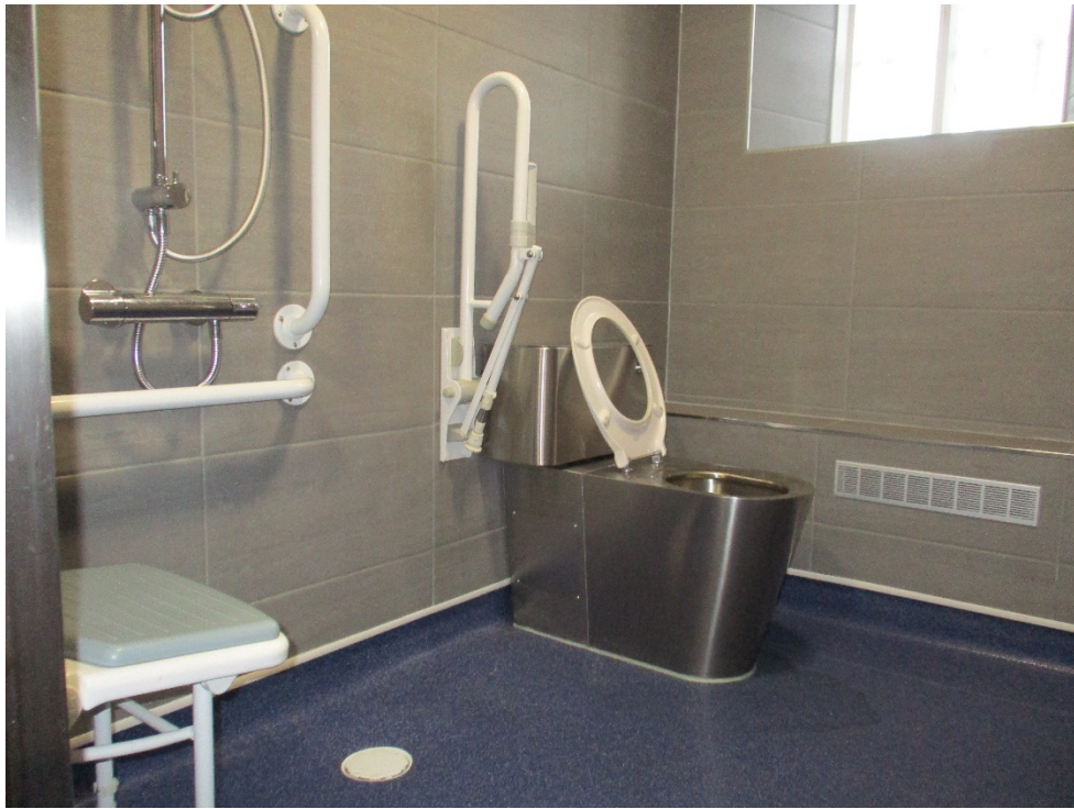
Wet room on F2 unit
