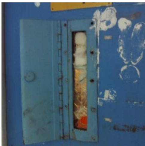
Damaged and blocked observation panel (left) and cell with broken window
