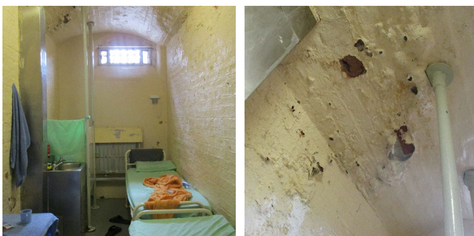
Mould and decaying paint in a cell on D wing
