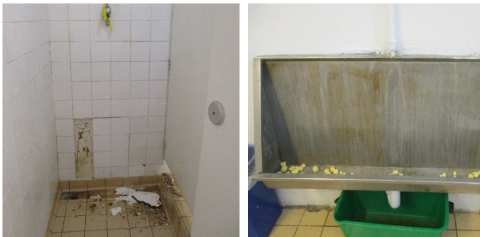
Shower with collapsed ceiling (left) and stained, leaking, smelly urinal on G wing
