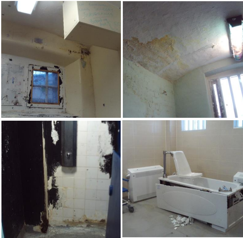
Damp and mould in cells (top row), shower cubicle (bottom left), and bathroom in the health care department (bottom right)
