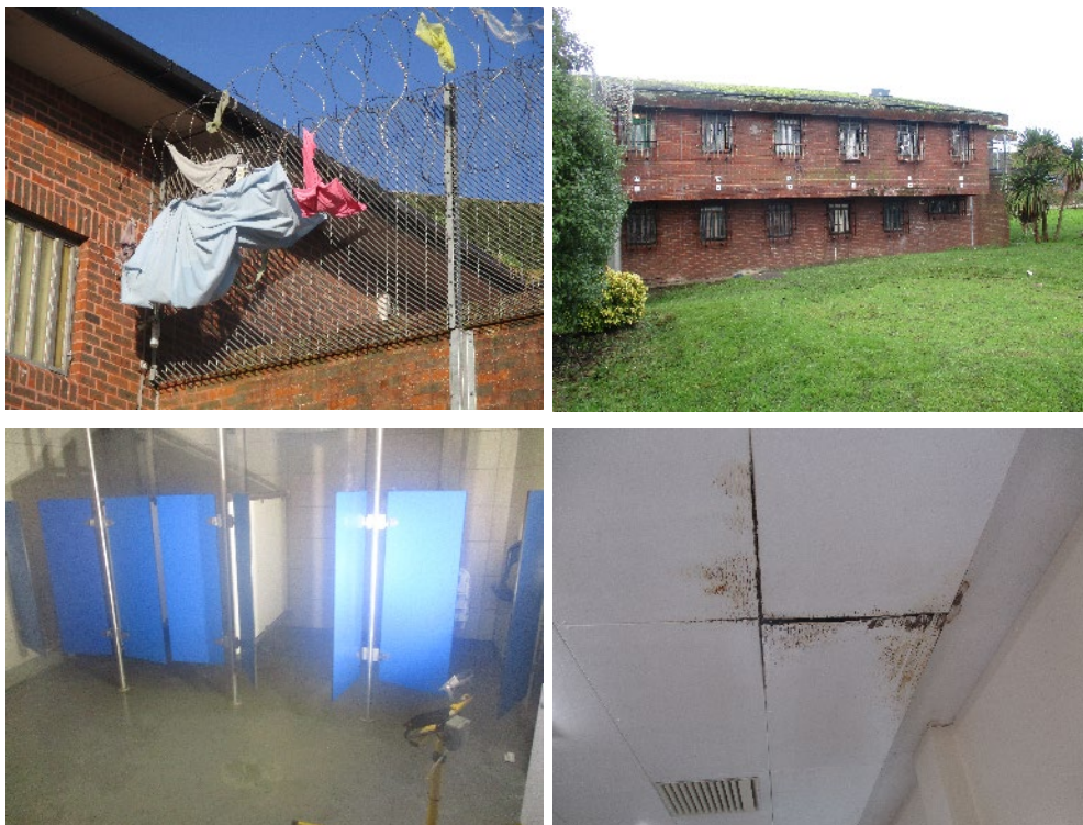
Two photos of the exterior of the unit (top), temporary lighting in showers (bottom, left), ceiling damage from leaking roof in gym (bottom right)
