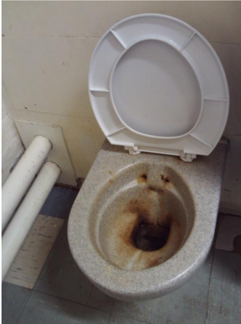
C wing cell toilet
