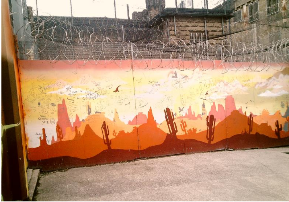
Low hanging razor wire in the segregation yard
