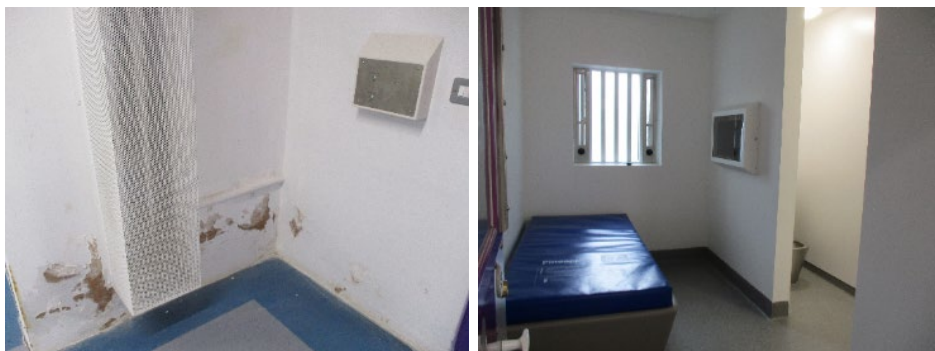
Cell awaiting refurbishment (left), and refurbished cell (right)
