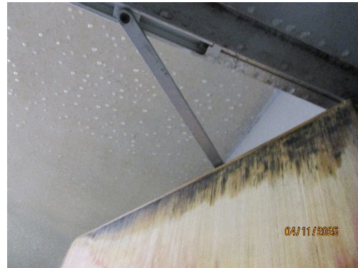
Floor in shower room on Dorset wing (left) and example of condensation and mould on Dorset wing
