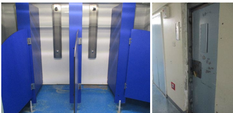
Showers on main residential house block (left); and peeling paint and missing plaster on main residential unit (right)
