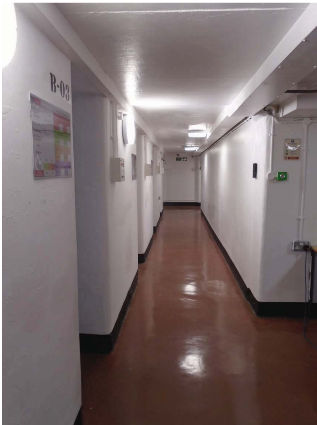
The refurbished segregation unit
