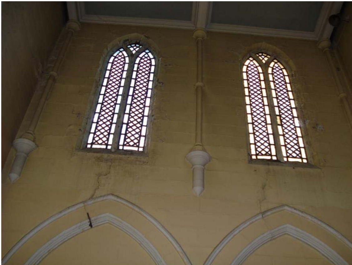
Water damage and structural defects in the chapel
